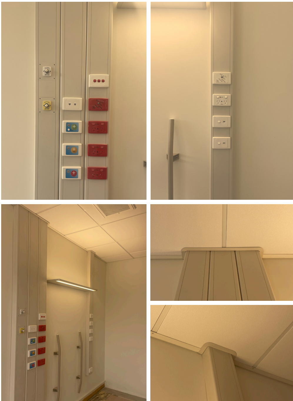
Images: Parkside Ward at Christchurch Hospital. Energylight 150v Trunking in two arrangements; one and three trunking in the system, either side of the bed head.
